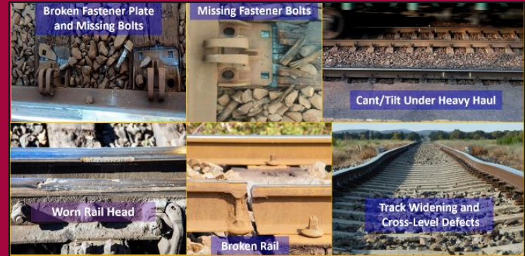
Track Integrity Monitoring System (TIMS) by Avante
